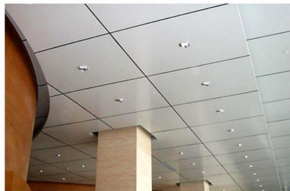
False Ceiling (Gypsum & Grid)
